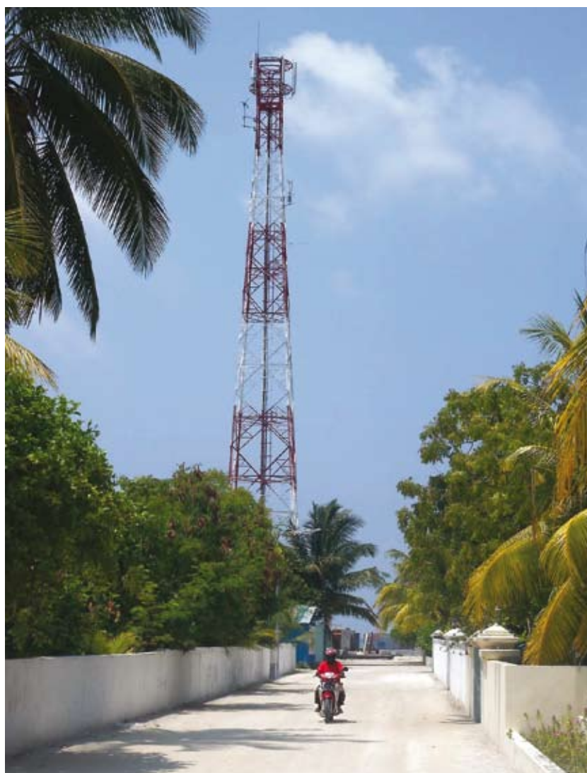
All inhabited Islands have coverage via antenna towers such as this, located on a main road in Gan-Fonadhoo, Laamu Atoll.
