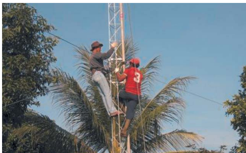
Radio tower being set up in Indonesia by KBR68H.
